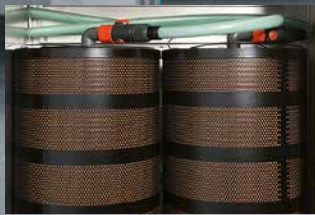
Filters For easy operation. We positioned the two filters side by side to make maintenance fast and easy.
